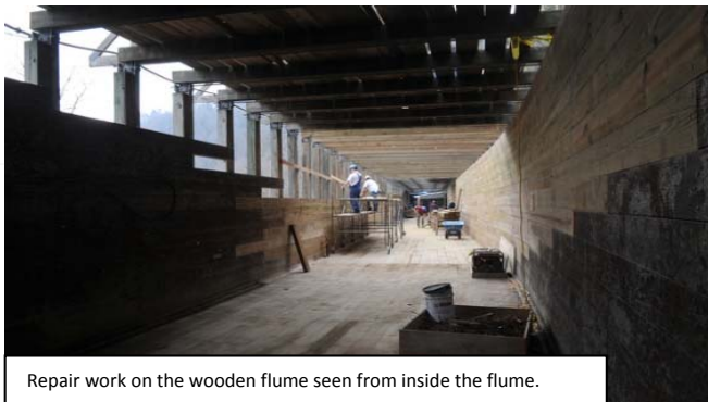
Where here it all begins. Ocoee dam #2 backs up the flow of the Ocoee River and diverts it to the powerhouse through a five mile wooden flume.
